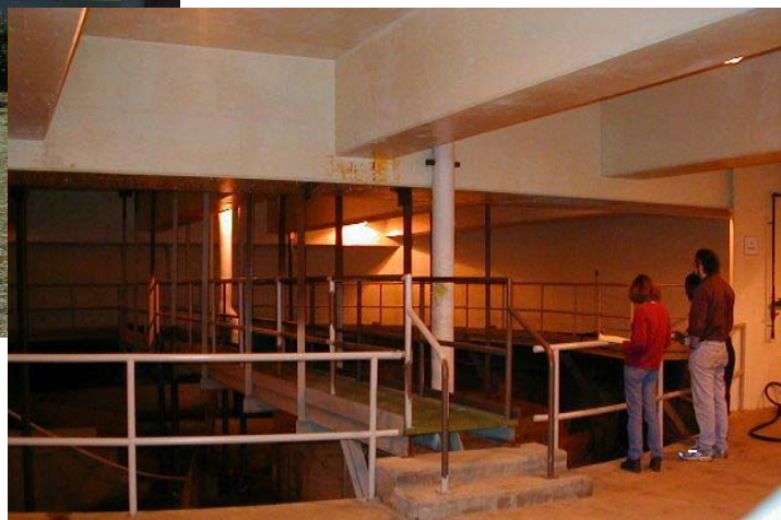
One of three 90 foot diameter separation tanks in the swirl concentrator facility
